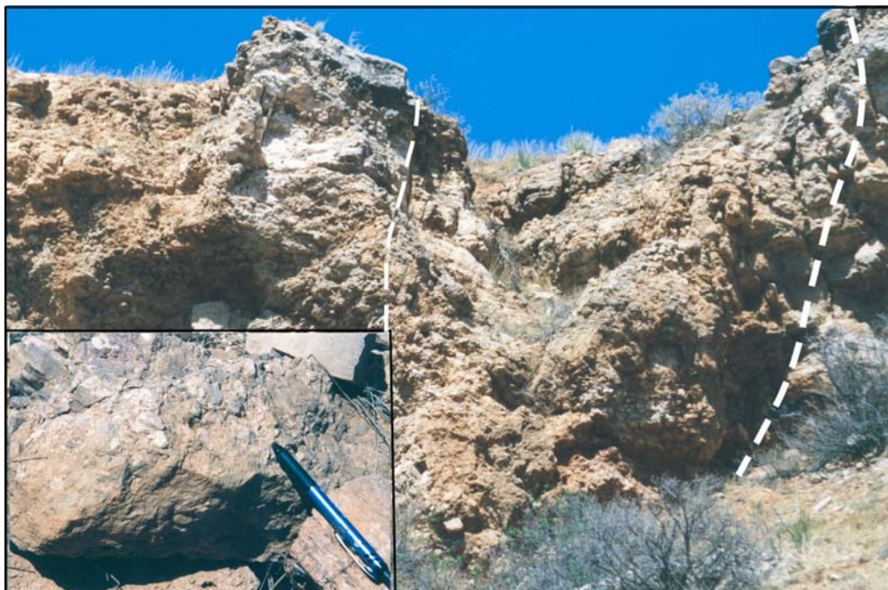
Figure 24. Collapse sinkhole (dashed line) in a zone of brecciated Minnekahta Limestone along Redwater Creek, one mile southeast of Stop 9. Inset shows details of breccia.
