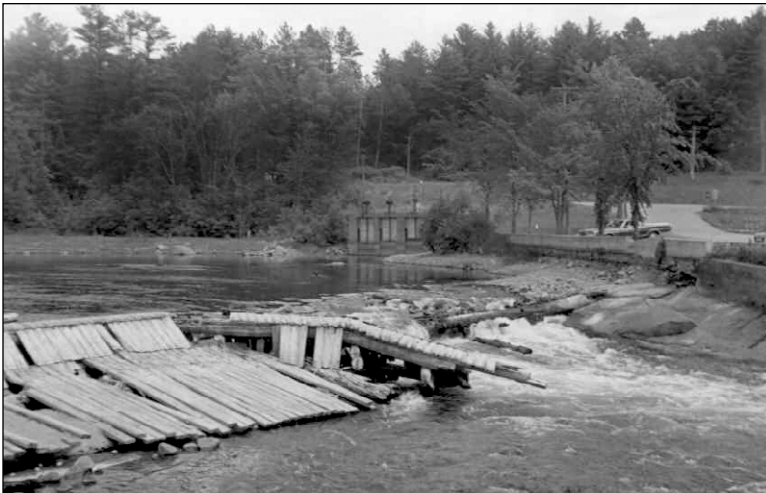
Figure 2. Photos of A , Balsam Row Dam in 1998, looking upstream at dam, B , Keshena Falls Dam in 1950, and C , failed Keshena Falls Dam, Wis., in 1972. (Photos B and C from the Wisconsin Department of Natural Resources, Dam File No. 72.1, Madison, Wis.)
