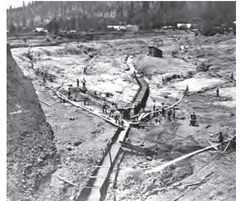
Figure 2. Gravel deposits were washed into sluices (from center to lower part of figure) where gold was recovered.
