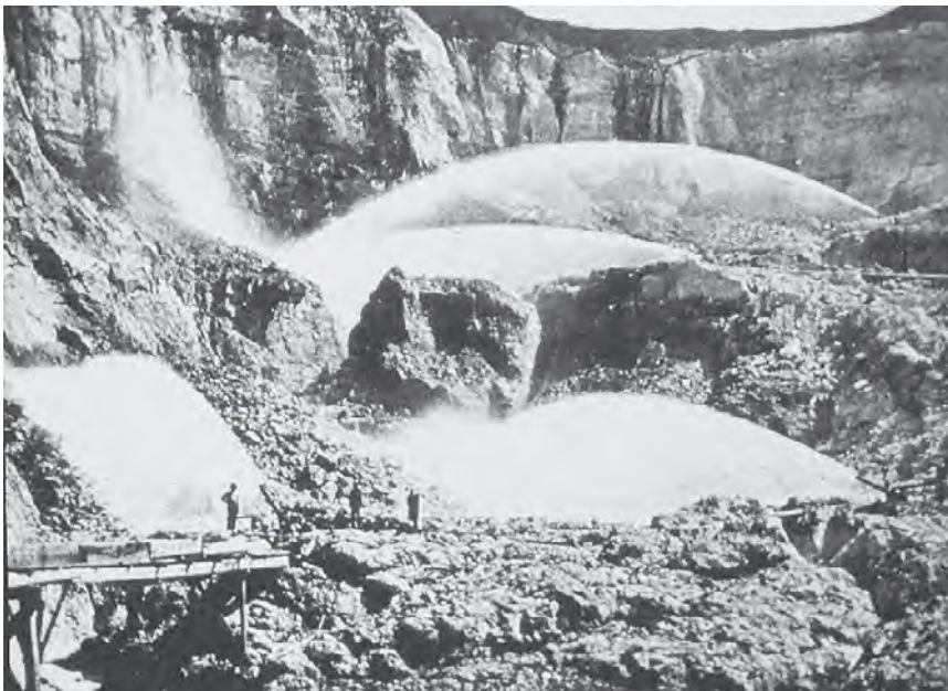
Figure 1. Monitors (water cannons) were used to break down the gold-bearing gravel deposits with tremendous volumes of water under high pressure. Some mines operated several monitors in the same pit. Malakoff Diggings, circa 1860.
