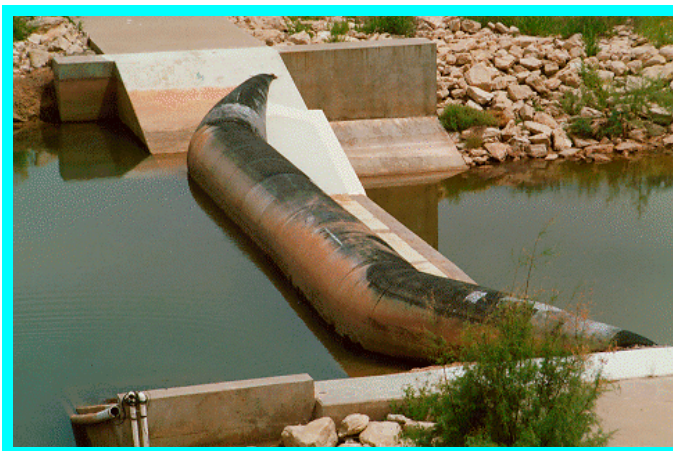
C. Water-control structure in Area VIII, Tex.
