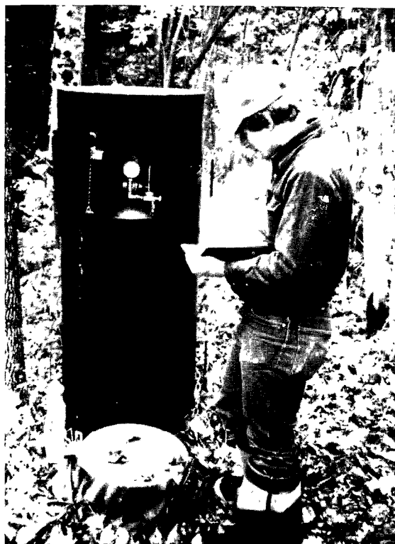
Figure 10.—One-hundred-pound propane gas cylinder inside protective circular steel housing; dual-stage regulator and flowmeter can be seen through access door on top of tank.
