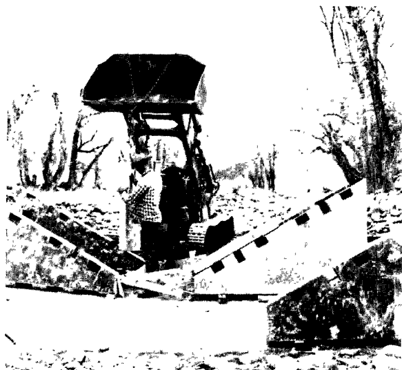
FIGURE 27.—Construction of 3-foot trapezoidal supercritical-flow flume using precast concrete components (note steel plates set in concrete to permit welding).
