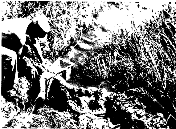
FIGURE 12.—Modified 3-inch Parshall flume installed for measuring discharge.
