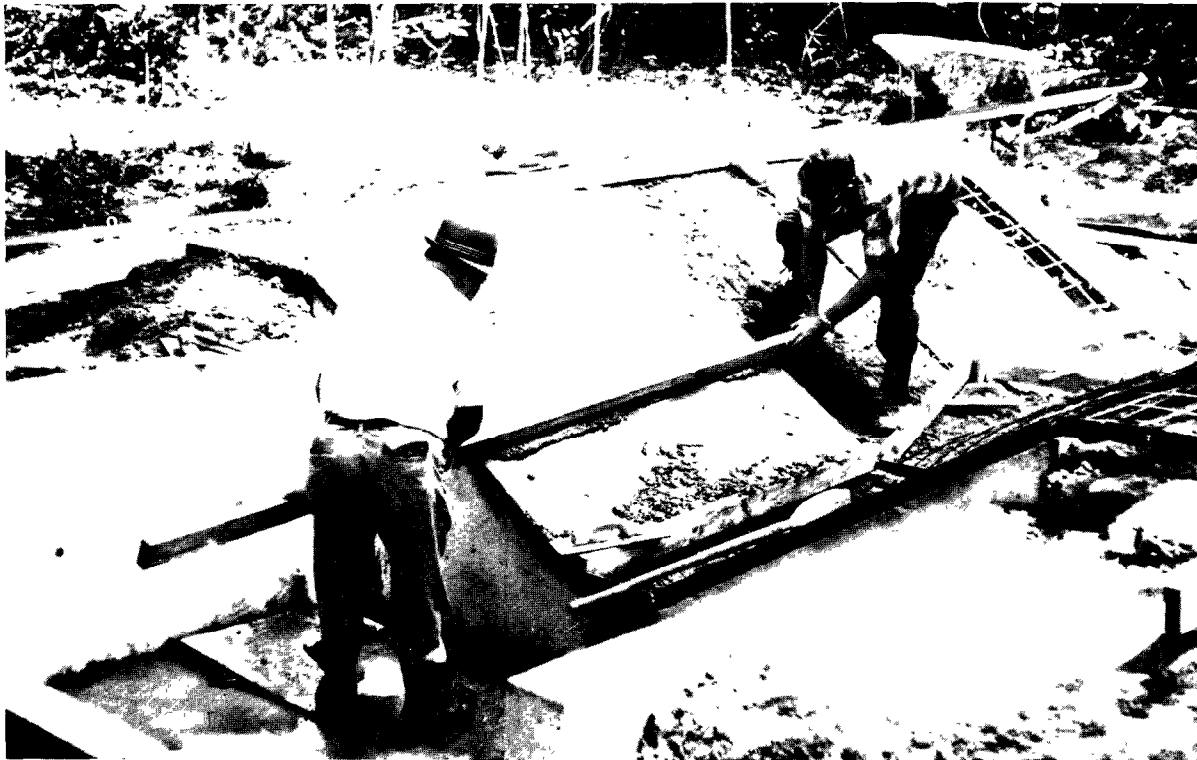
FIGURE 33.—Concreting of throat section of 1-foot trapezoidal supercritical-flow flume using steel angle screeds.
