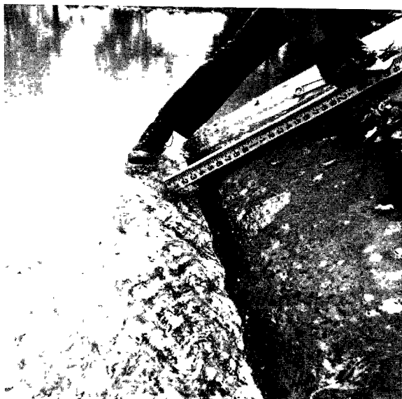
FIGURE 23.—Erosion of concrete on floor and walls of the throat of a trapezoidal flume.
