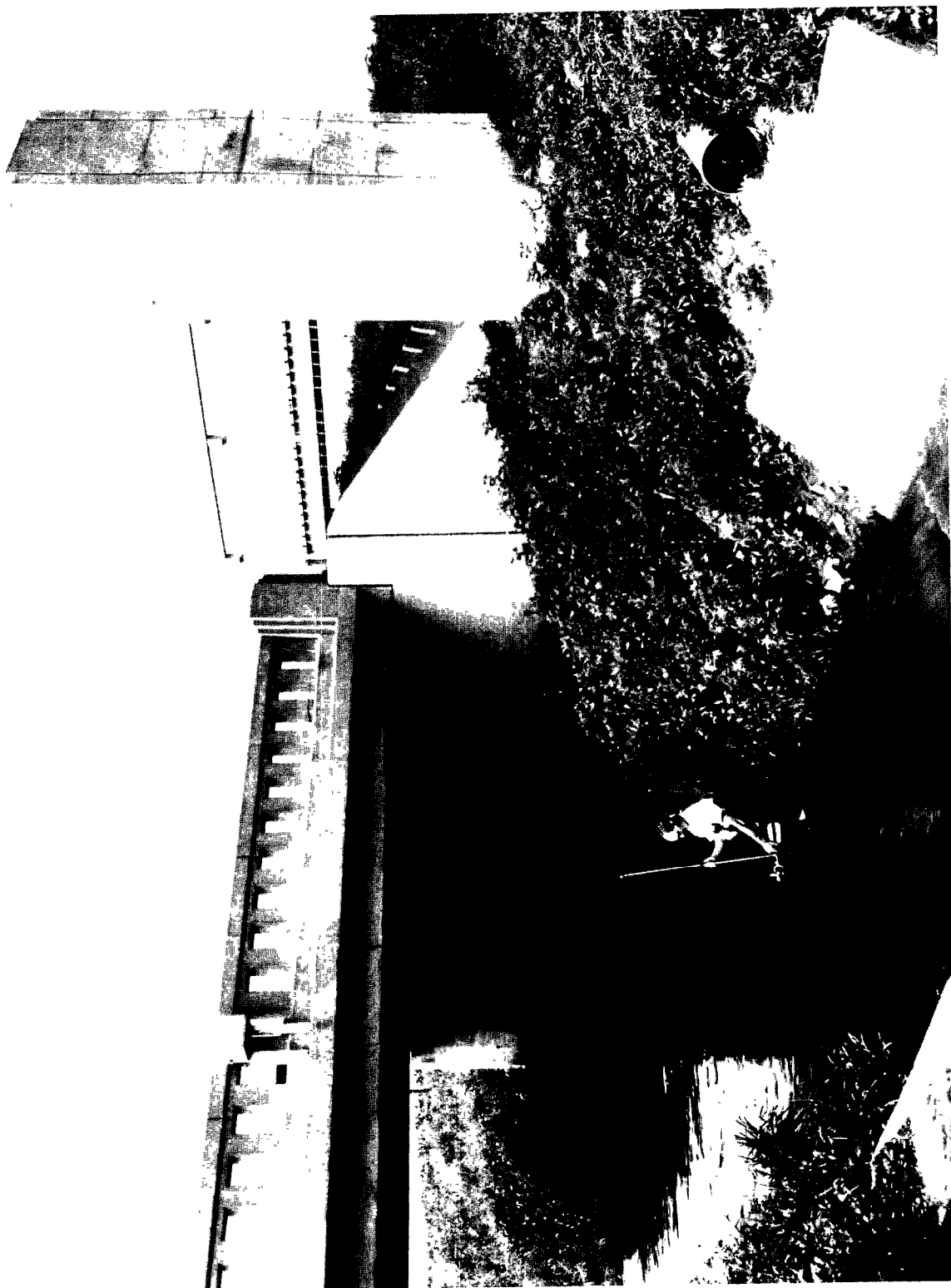
Figure 2.—Gage, concrete control, outside gage on bridge, and an engineer making a wading measurement, Kaskaskia River at Bondville, Ill
