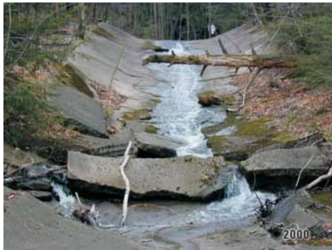
Figure 3. View of mine refuse blocking Nanticoke Creek upstream of Leuder Creek, Luzerne County, Pennsylvania.
