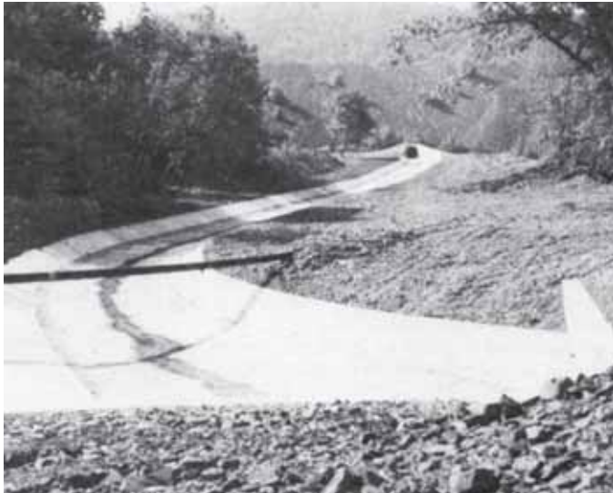
Figure 2. View of a concrete flume built in 1958 to minimize infiltration of Leuder Creek into the underground mine workings, Luzerne County, Pennsylvania. Photograph from Dierks and others (1962).
