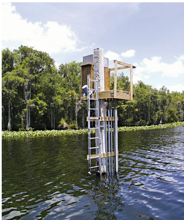
Figure 5. Data-collection structure at the Suwannee River above Gopher River data-collection site.
